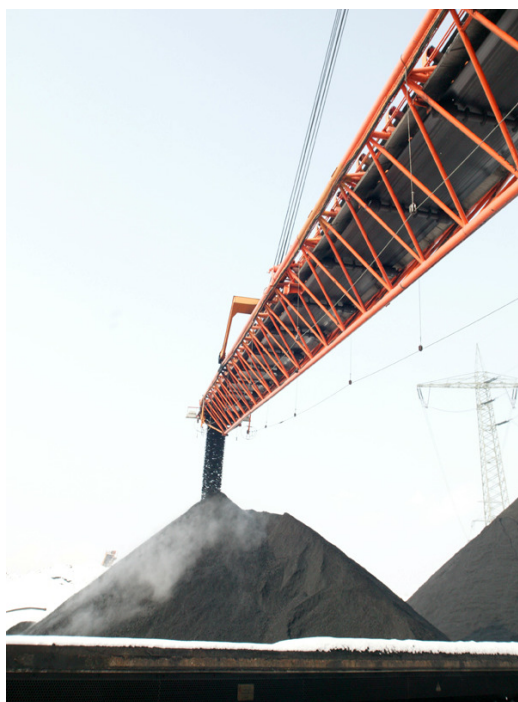
Coal-fired power plant in Scholven
